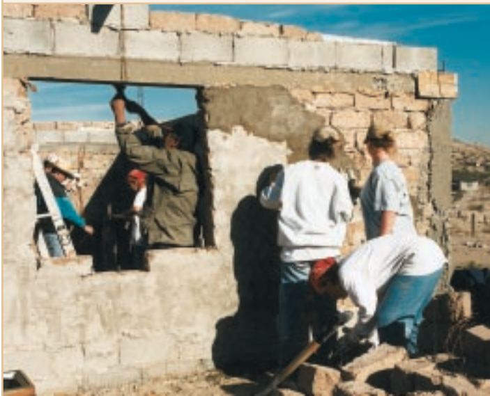
Walls are made from adobe bricks and sealed on the outside with stucco.
